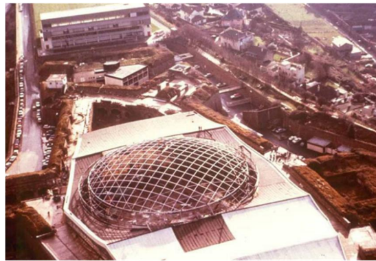
Single layer steel levic dome in Fort Regent leisure centre, diameter 58 m, Jersey
