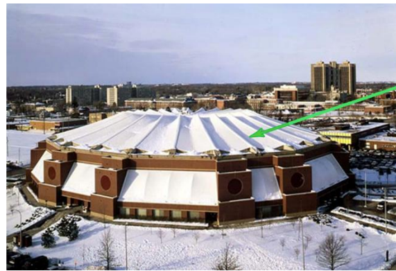
Redbird Arena, elliptic cable dome at the Illinois State University, 78 m × 93 m, height 24m, central part of the dome has a dip, capacity around 10000, type of membrane cover: PTFE coated glass fibre fabric, Illinois, USA, 1988, Geiger Engineering
