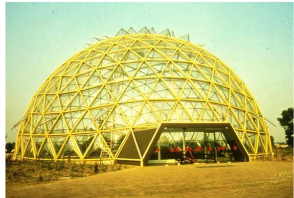
Green house, single layer steel geodesic dome with rigid acrylic cladding panels, 36 m diameter, Düsseldorf, Germany, Mero
