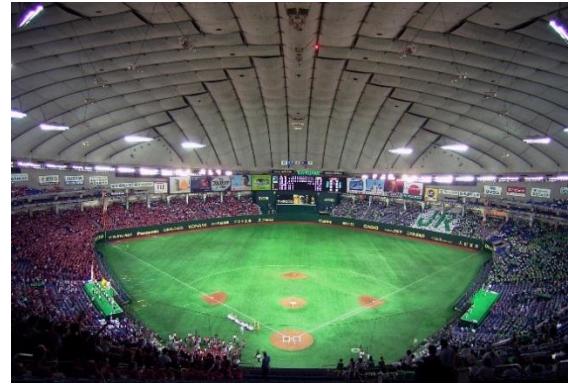
Tokyo Dome (Big Egg), multipurpose air-supported cable reinforced membrane structure, span: 200 m, Tokyo, Japan, 1988, Takenaka Corp, Nikken Sekkei
