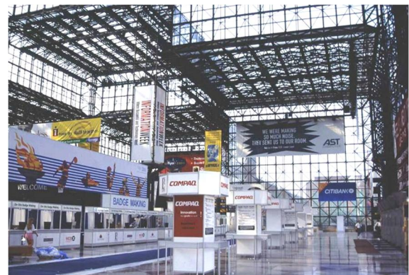
Jacob K Javits Convention Center of New York, USA, provides total exhibition area of about 90000 m 2 , consists of double layer grids for roof, floors and walls, 1986
