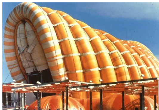
Air supported membrane structure, contractor's field office, Japan
