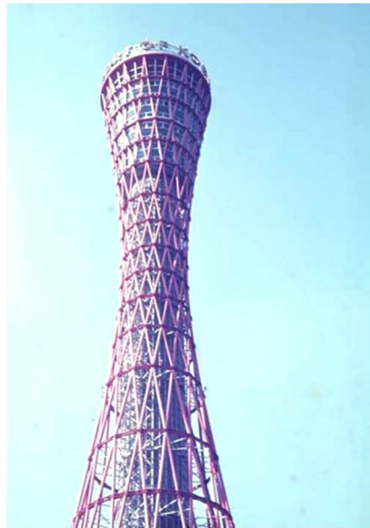
Tubular steel hyperboloidal television tower, Kobe, Japan
