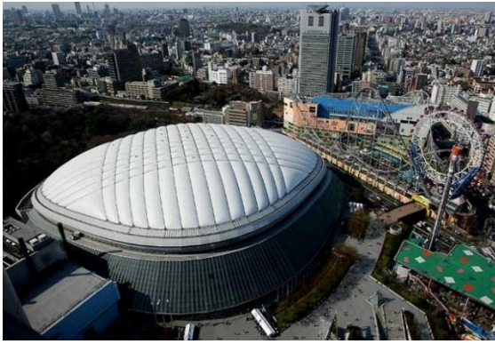
Tokyo Dome (Big Egg), multipurpose air-supported cable reinforced membrane structure, span: 200 m, Tokyo, Japan, 1988, Takenaka Corp, Nikken Sekkei
