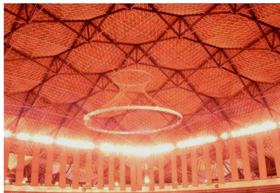
Spatial structure roof involving hyperbolic paraboloidal parts (hypars), Mexico, Felix Candela
