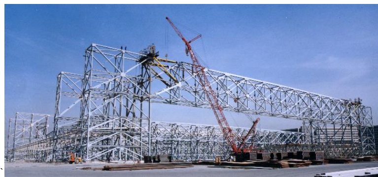
Tehran overhaul Hangar, plan: 196×200 m, span: 156 m, height: 35 m, MSA, Namvaran, SAFIRA, M Heristchian, 1998
