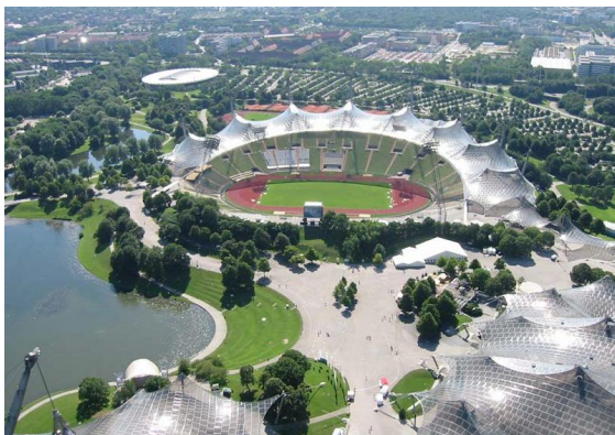
Munich Olympic stadium cable structures, built for the Olympics 1972, Munich Germany, Frei Otto, Jörg Schlaich
