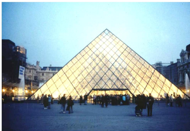
Louvre museum courtyard, double layer pyramid with stiff elements and cables, Paris, France
