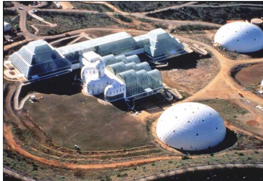
Pyramidal spatial structure (and other forms: including two geodesic domes and three stepping barrel vaults), astronaut training center, Nevada, USA, Peter Pearce
