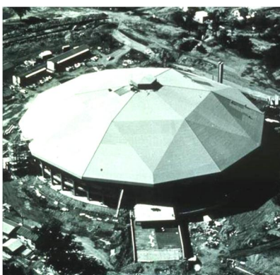
Makomanai Olympic skating stadium, faceted dome with a span of over 100 m, Japan, Tomoe Corp
