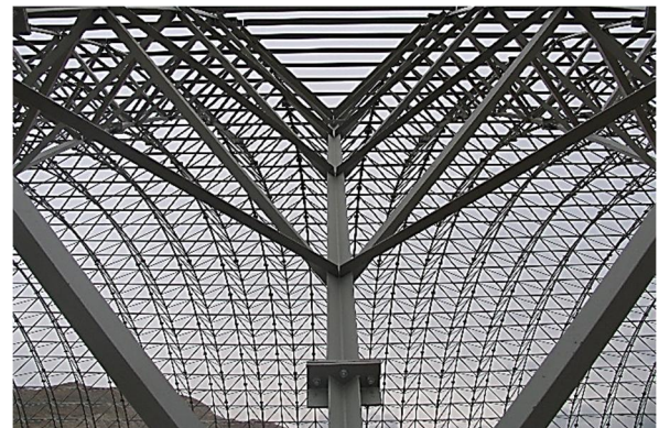
Sufian cement factory material store, span: 67 m, length: 201 m, Iran, Tabriz, Sufian, 2006, M Heristchian, Porsaz Co
