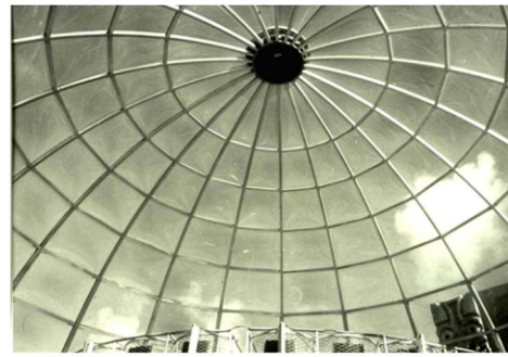
Tubular steel ribbed dome, New Delhi, India
