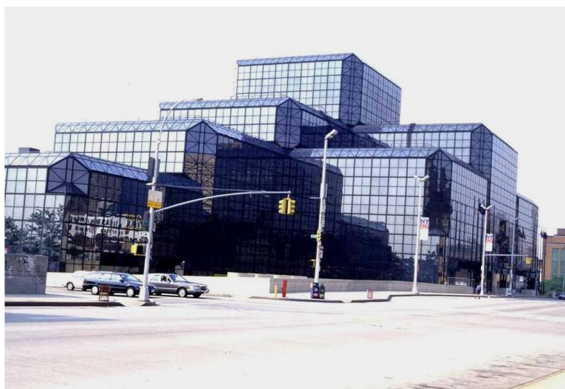
Jacob K Javits Convention Center of New York, USA, provides total exhibition area of about 90000 m 2 , consists of double layer grids for roof, floors and walls, 1986
