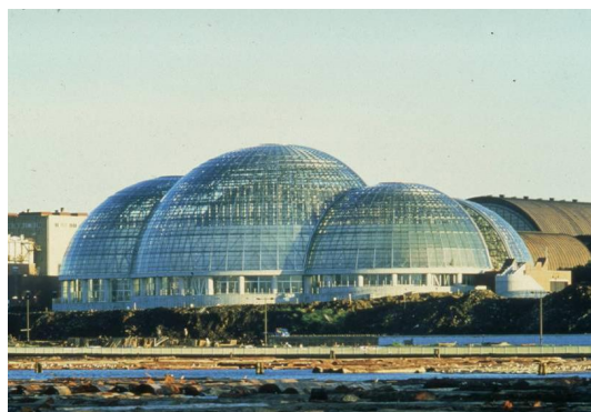
A compound dome for a greenhouse, Japan, Tomoe Corp
